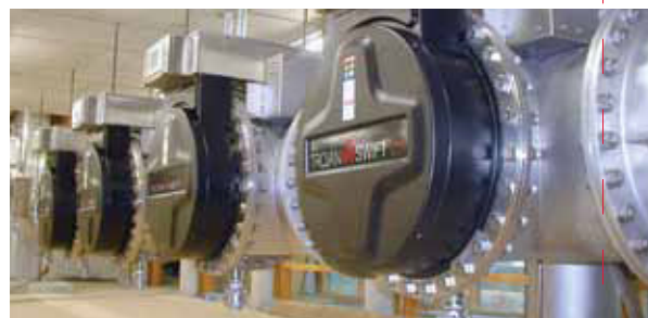
A TrojanUVSwift™ECT system installed at the PWN Water Supply Company in Andijk, the Netherlands.
